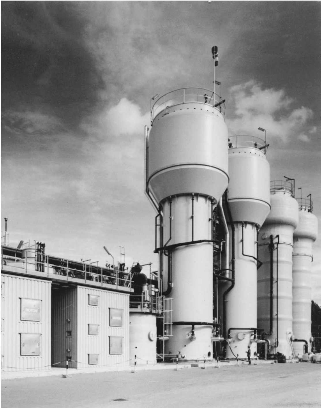
Figure 10. View of an industrial anaerobic wastewater treatment plant based on the operation of fluidized-bed reactors, Gist-brocades, Delft, The Netherlands. Source: From Ref. 34.
